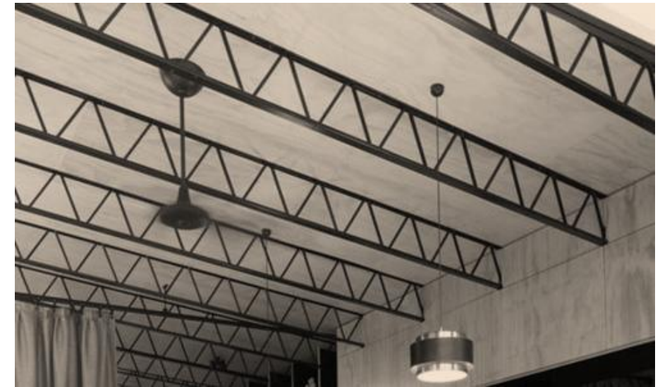
4. STEEL TRUSSES WITH SUSPENDED LIGHTS
